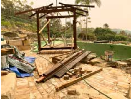
The tea house framed up.
