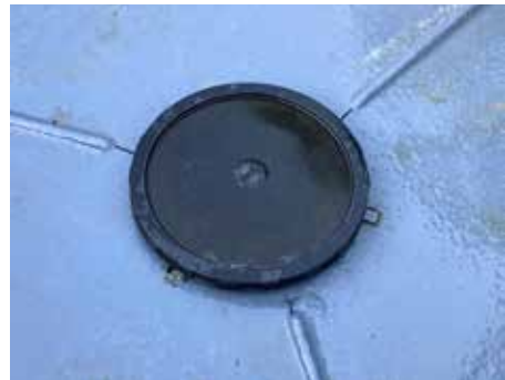
New bottom drain for larger koi can be removed to allow fry insert for newly hatched fry.
