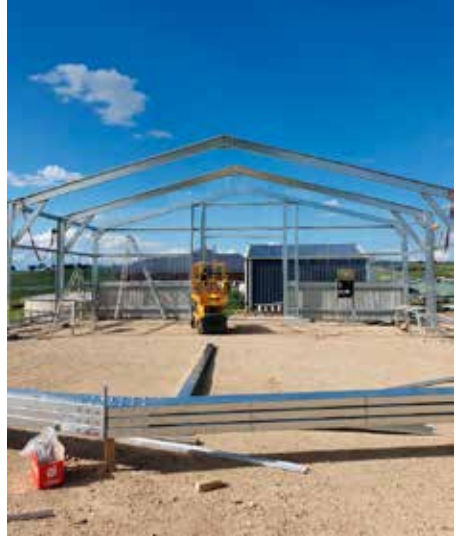
Shed pad complete and erecting the new fish house begins.
