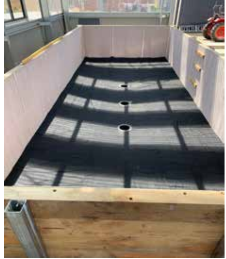
The main Pond ready for the liner to be installed.
