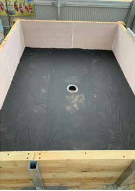
Breeders pond, ready for the liner to be installed.
